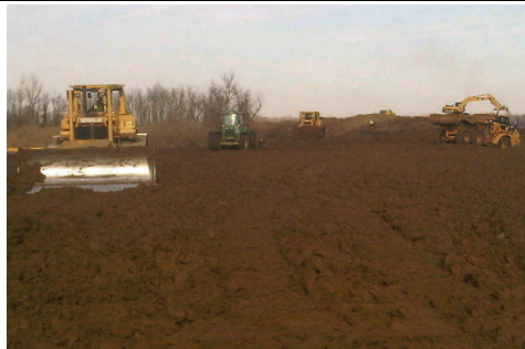
Crews reconstruct the levee at the center crevasse Friday. Earthwork resumed Thursday afternoon.
